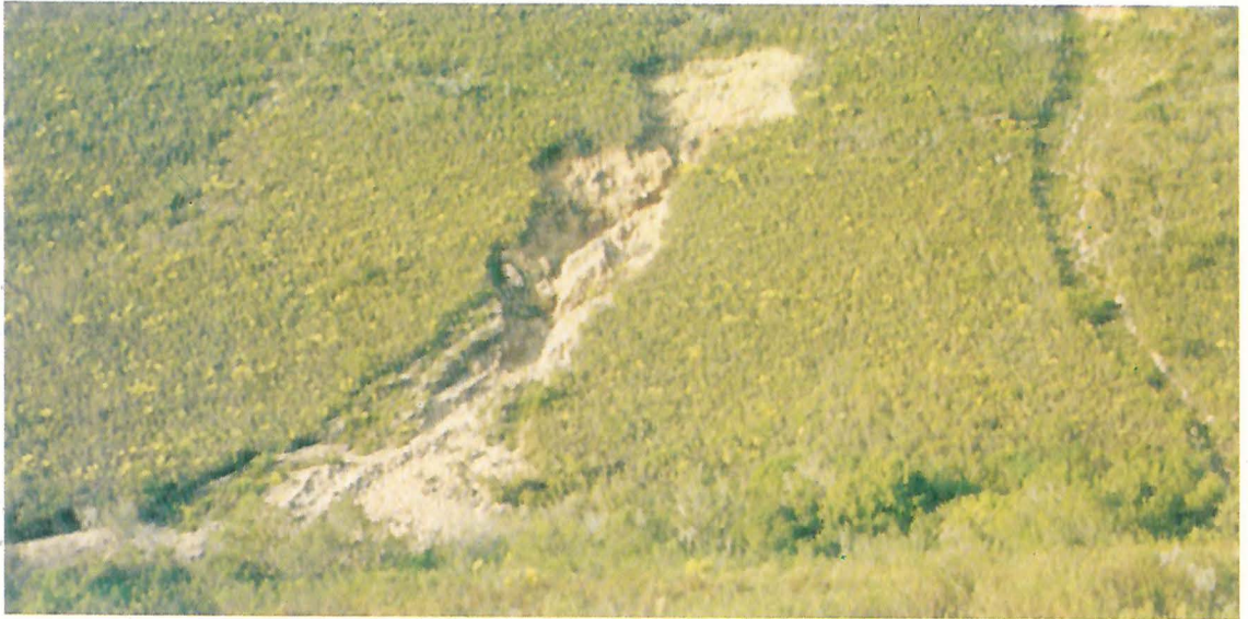
Figure 2.4: Soil erosion in drainage region L9.
