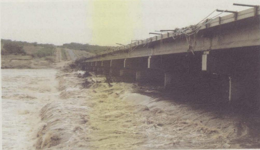
46. Great Usutu River: downstream side of bridge on the Manzini-Mahamba road with submerged low-water bridge, upstream of Site 47 (C.J. Rodda)
