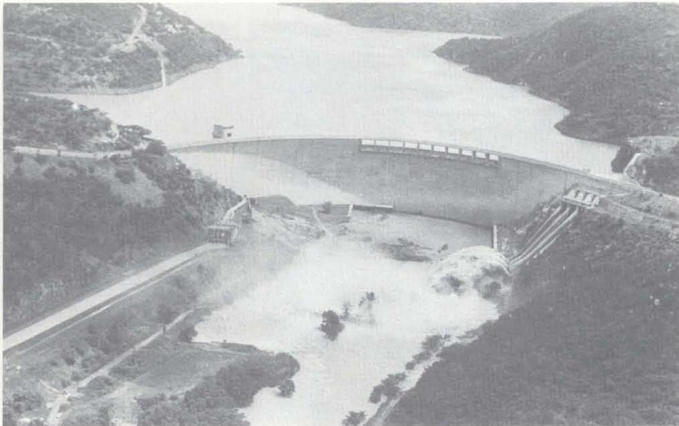
41. Pongolapoort Dam: general view during flood release of  $\sim 1\,000\text{ m}^3/\text{s}$  on 8 February 1984, Site 32
