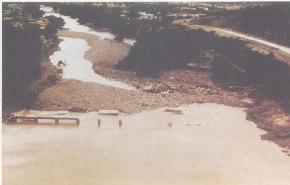
42. Pongolapoort Dam: downstream view of jet plunge pool with damage caused by release, Site 32
