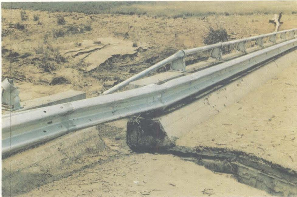
24. Mkuze River: downstream close up picture of damaged N2 road bridge deck
