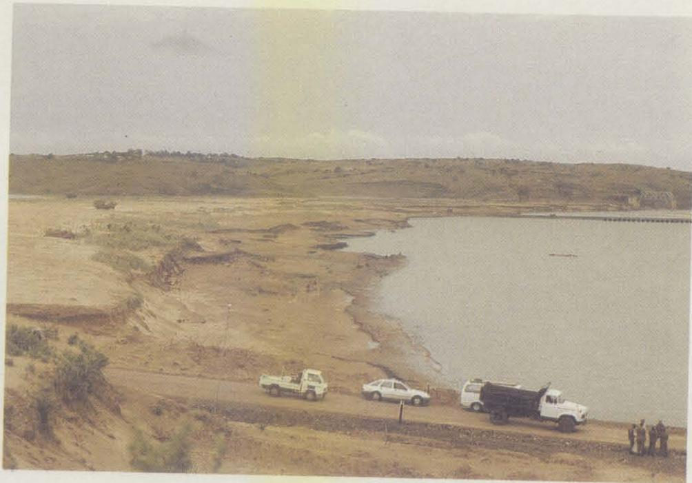
19. Mfolozi River: erosion and deposits along left bank downstream of the N2 road bridge
