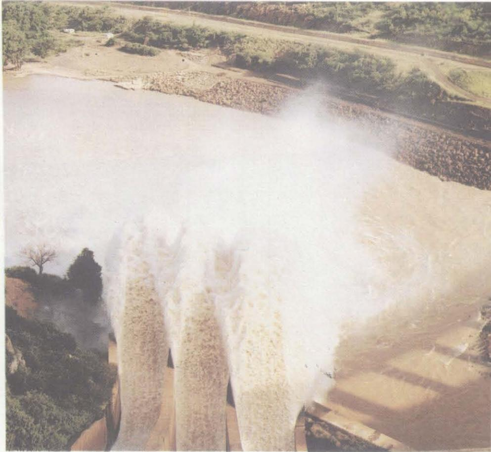
43. Pongolapoort Dam: testing of modified chutes with a release of  $400 \text{ m}^3/\text{s}$  and rip-rap protection of damaged right-bank, Site 32 (D.R. Clark, Engineer, Department of Water Affairs)
