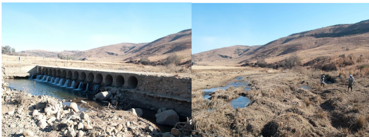
Figure 58. Poor design of the stream crossing ensures the blockage of fish movement, especially during low flow conditions. The deposition of sediments above the crossing (photo on right) covers the substrate for approximately 200 m (08 July 2015, G Diedericks).
