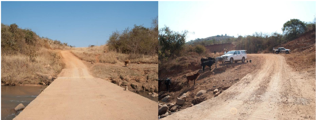
Figure 96. The road approach from both sides of the stream is steep with no drainage. Loose soil from the road enters the river directly during rainfall events (05 August 2014, G Diedericks).
