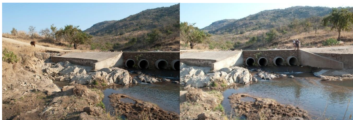
Figure 145. Bank scouring (left photo) downstream from crossing as it overtops during high flow events. The crossing (right) block fish movement during normal and low flow events (05 August 2014, G Diedericks).
