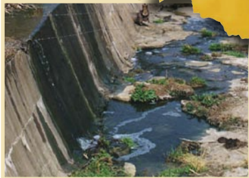
Raw sewage overflows into rivers where sewage treatment works are not upgraded timeously, or are operated inefficiently, such as here near De Wetsdorp.
