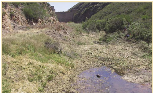
The Hartenbos River has stopped flowing downstream of the Hartebeeskuil Dam due to the lack of water release mechanisms.
