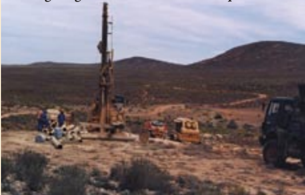
Drilling for groundwater in the Namaqualand
