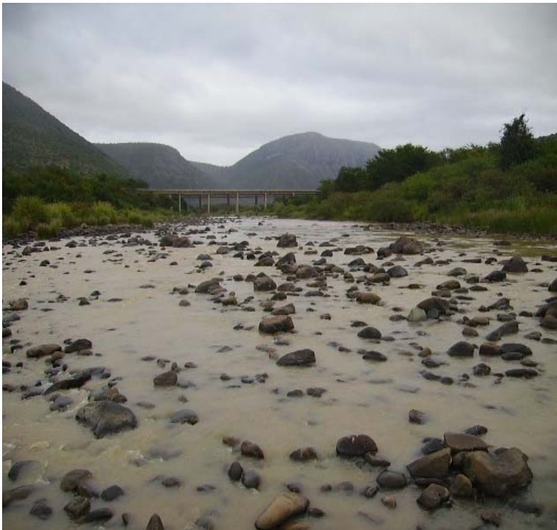
Plate 12. Kei River bridge site.
