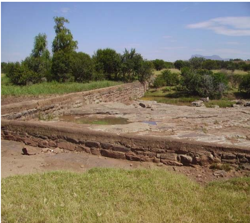
Plate 3. The river was no longer flowing and a weir was designed to collect any droplet of the water.
