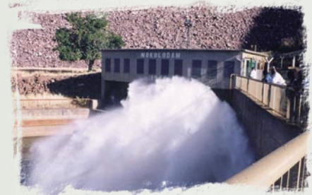
Mokolo Dam sluice gates
