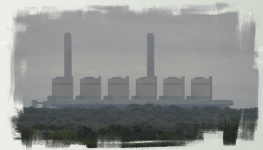
Matimba Power Station
