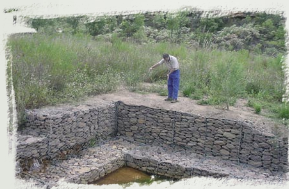
Examining a rock gabion
