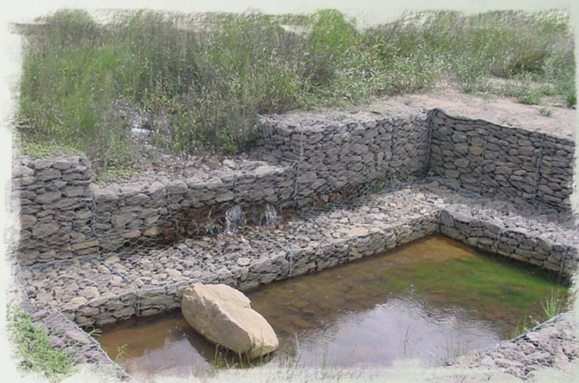
A rock gabion, showing the structure and the water flow
