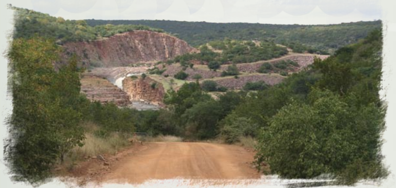
View towards the Mokolo Dam outflow
