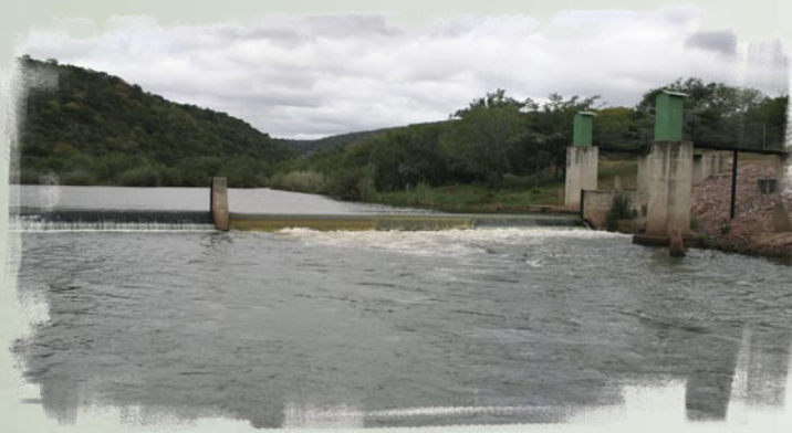
Gauging weir below Mokolo Dam
