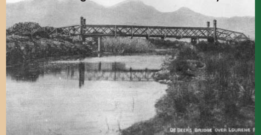
Lourens River bridge
