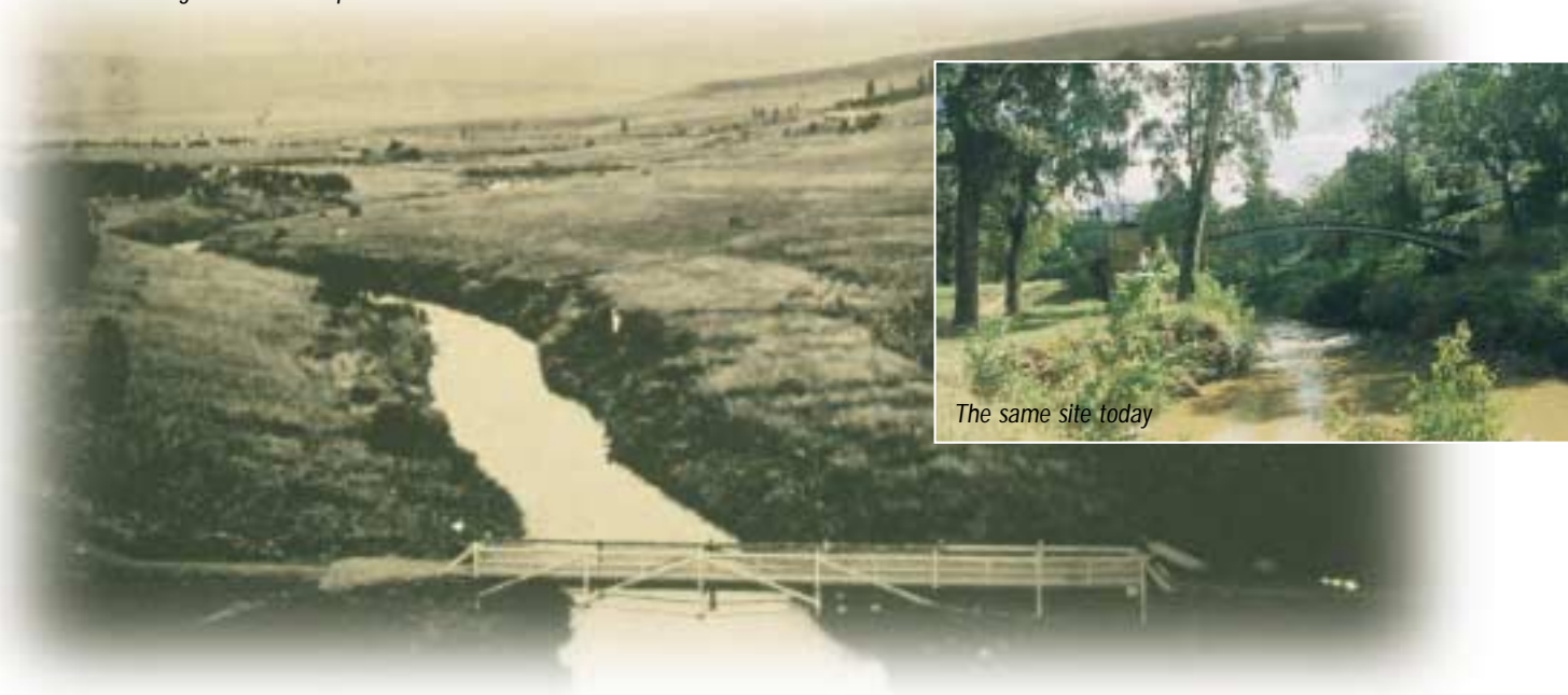
Footbridge between Chapel Street and Alexandra Park - 1866
