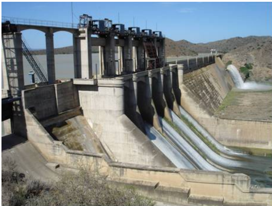
Figure 3.4 Darlington Dam on the lower Sundays River
