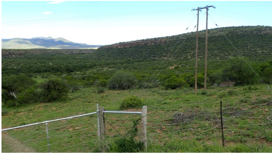
Figure 8: Photograph of existing power line along MR00639
