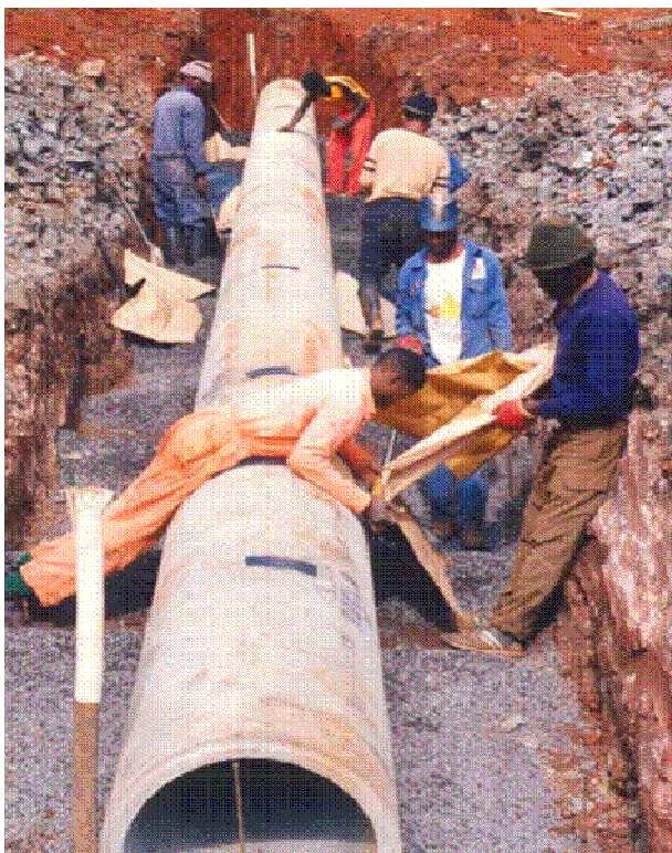
Figure 3.13: Pipe laying
