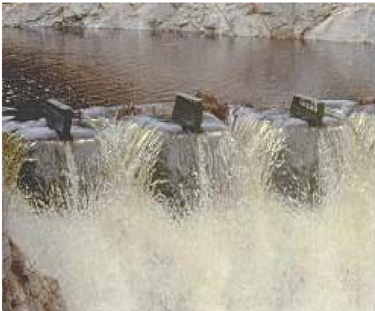
Figure 3.2: Operational Fuse gate
