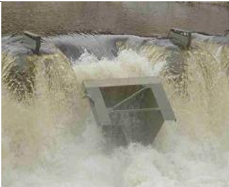
Figure 3.3: A Collapsing fuse gate
