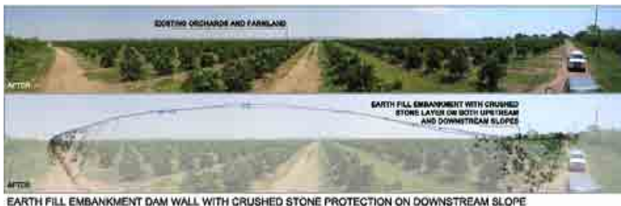
Figure 9.3: Erection of proposed new dam wall
