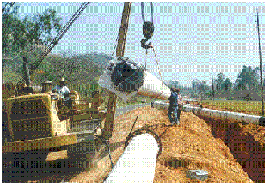
Figure 3.14: Trench for pipe laying
