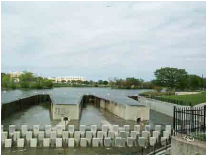
Figure 3.5: Example of a labyrinth Spillway (the “teeth” downstream are used to break the energy of the water and prevent erosion)
