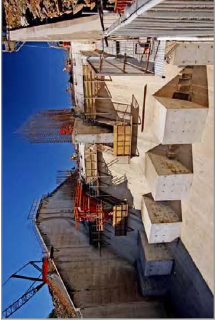
PHOTO OF ROSS RIVER DAM SPILLWAY DURING INSTALLATION OF FUSEGATES
