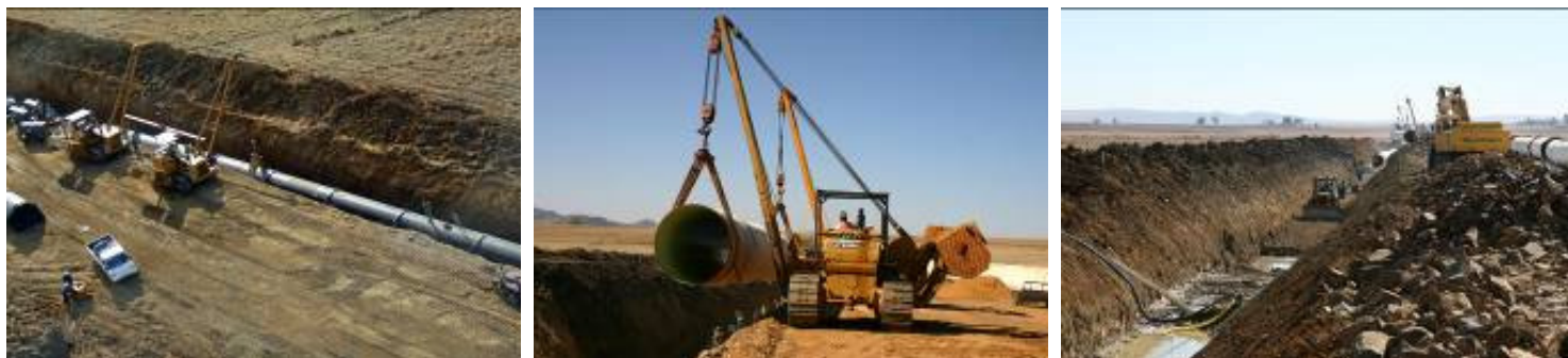
Figure 17: Typical trench excavation and pipe installation activities
