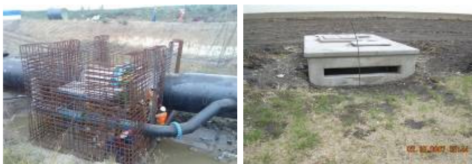
Figure 18: Typical examples of chambers (left - during construction; right – completed)
