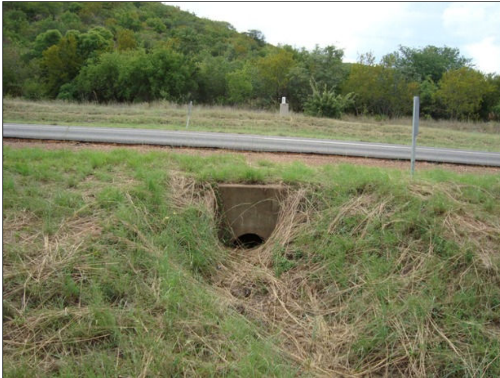
Figure 5: Drainage channels where the proposed pipeline alignment occurs alongside a roadway, which incorporated culvert drains that allowed for free drainage of water within the road reserves.
