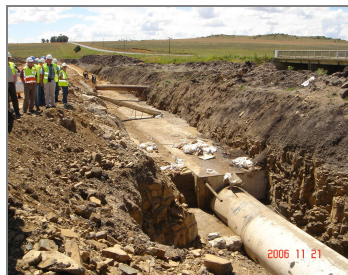
Figure 7: Typical river crossing showing concrete encased pipe section
