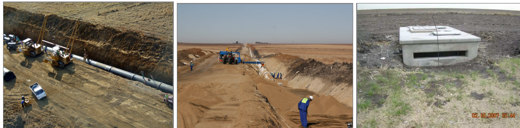
Figure 6: Typical trench excavation and pipe installation activities
