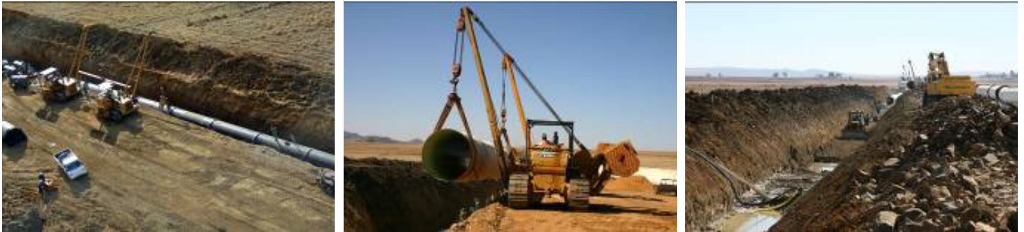
Figure 6 - 1: Typical excavation and pipe laying activities
