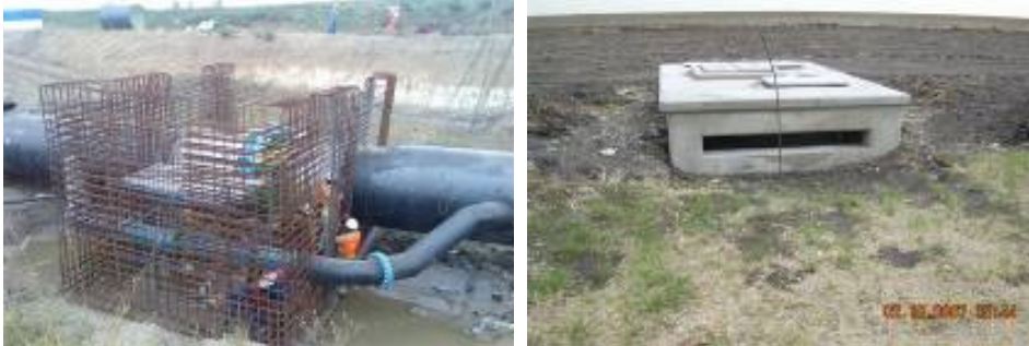
Figure 6 - 2: Access chamber during construction and once complete
