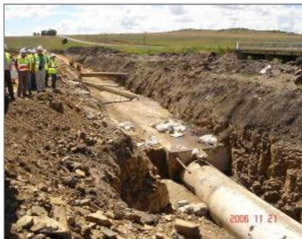
Figure 20: Typical river crossing showing concrete encased pipe section
