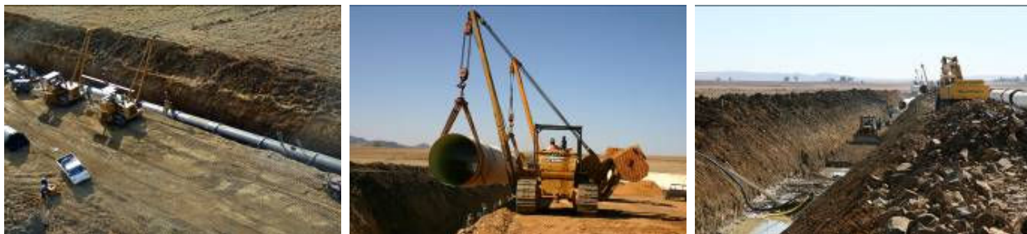
Figure 17: Typical trench excavation and pipe installation activities
