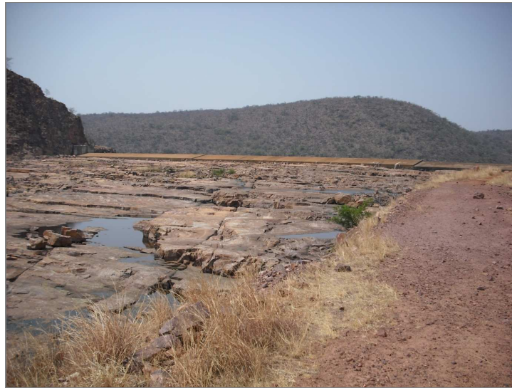
Figure 19: Crump weir and rock spillway at Mokolo Dam
