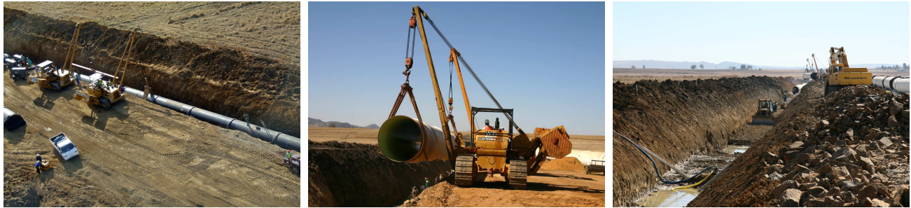
Figure 15: Typical trench excavation and pipe installation activities
