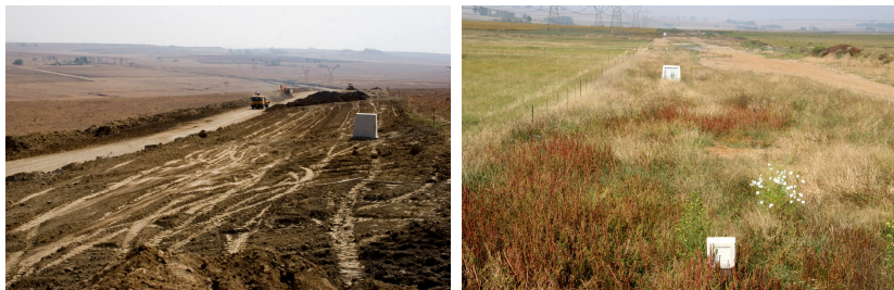
Figure 17: Typical views of reinstated (left) and rehabilitated (right) pipeline routes
