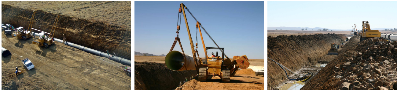
Figure 15: Typical trench excavation and pipe installation activities
