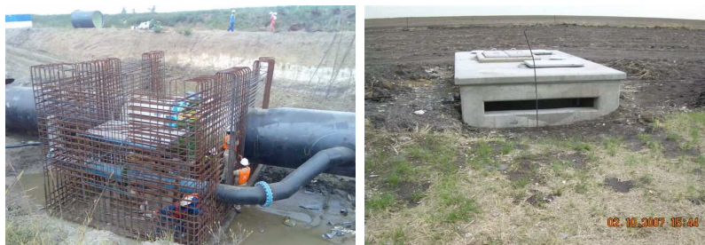
Figure 16: Typical examples of chambers (left - during construction; right – completed)
