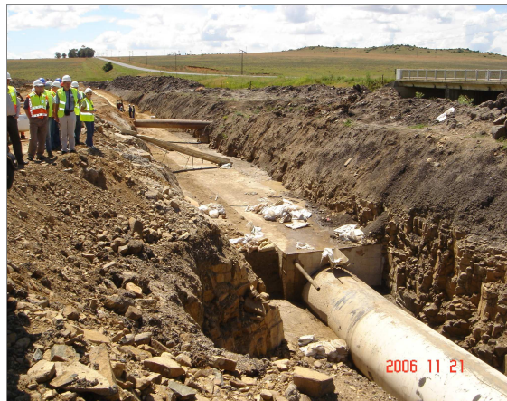
Figure 18: Typical river crossing showing concrete encasement pipe section
