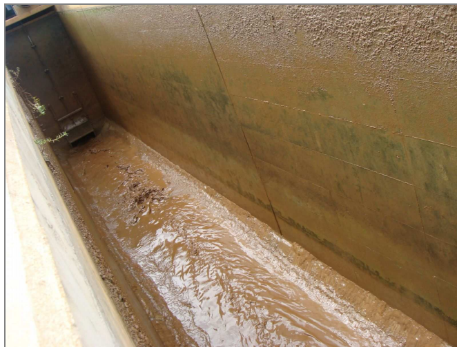
Figure 18: A view of the inside of a desilting channel at Lebalelo Weir Desilting Works (example)
