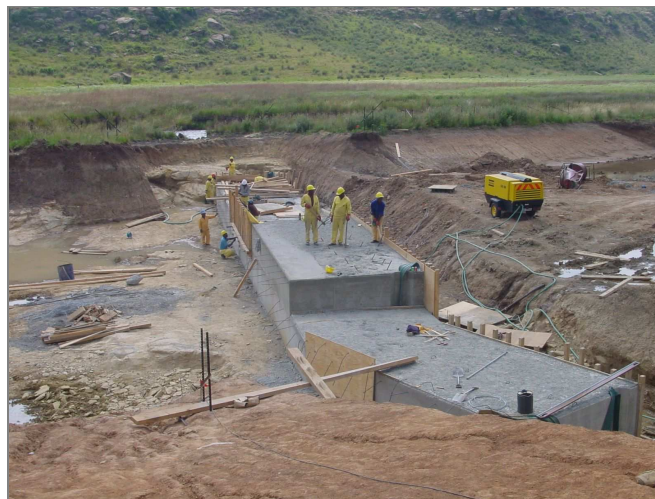
Figure 12: Example of construction of mass concrete weir structure (on Ash River) in progress
