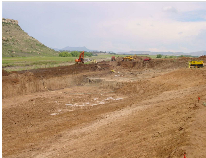
Figure 11: Example of site clearance and earthworks in progress (weir on Ash River)
