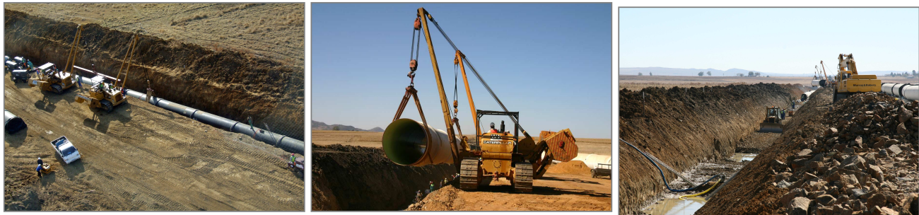
Figure 34: Typical trench excavation and pipe installation activities
