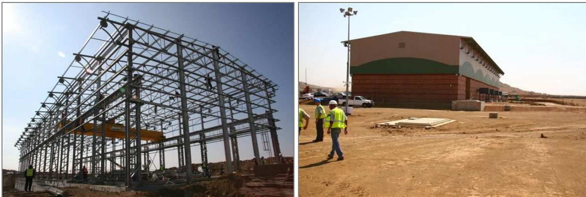
Figure 23: Steelwork and completed structure for a High-lift Pump Station (example)
