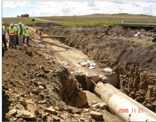
Figure 37: Typical river crossing showing concrete encasement pipe section
