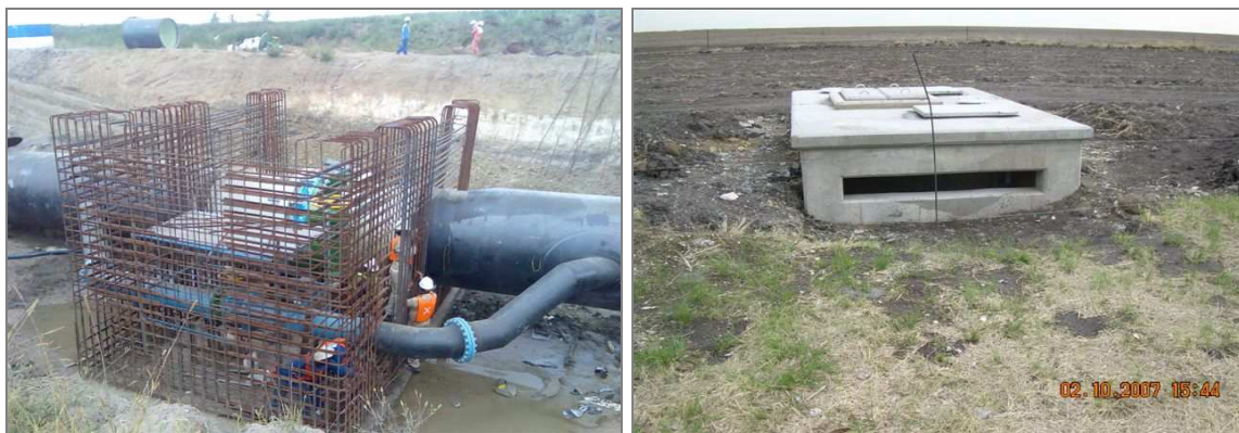
Figure 35: Typical examples of chambers (left - during construction; right – completed)
