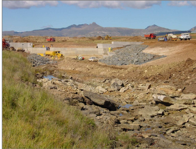
Figure 13: Example of downstream rip-rap protection placement (weir on Ash River)
