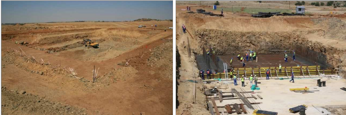
Figure 22: Excavation (left) and foundation (right) for a High-lift Pump Station (example)
