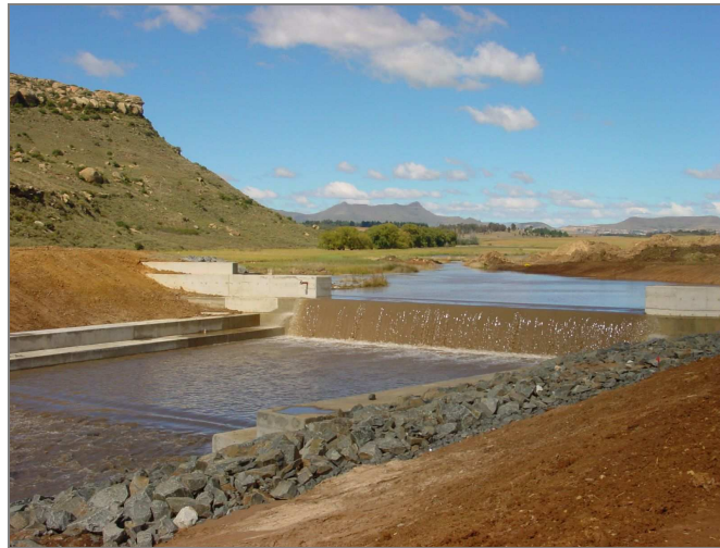
Figure 14: Example of weir structure (on Ash River) soon after completion
