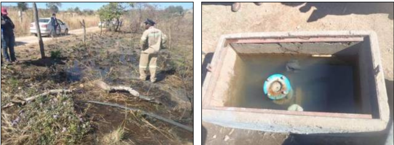
Figure 6.2: Leaking illegal connection and air valve
