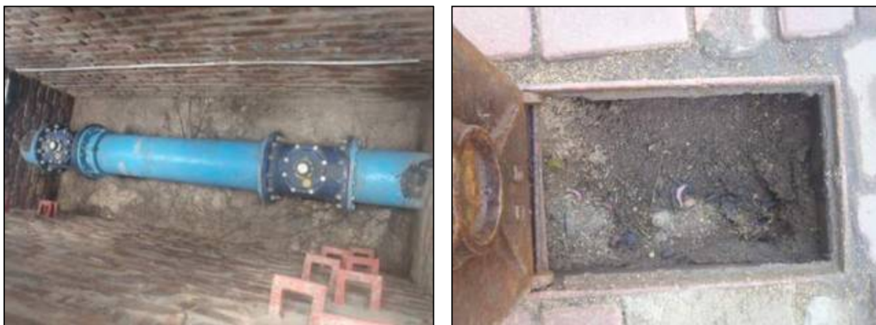
Figure 4.1: Bulk meter and buried consumer meter
