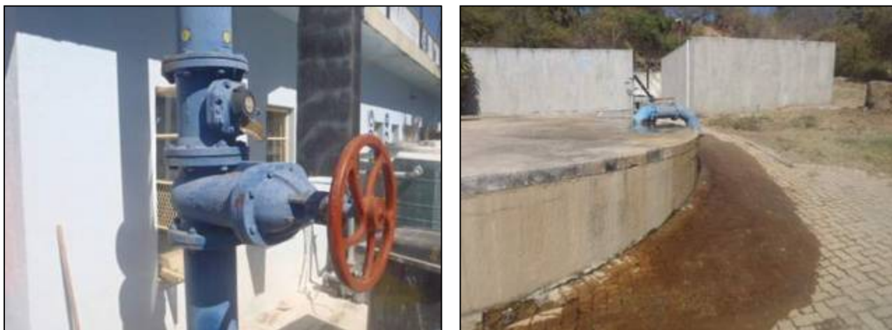
Figure 5.1: WTW inlet meter and leak at balancing reservoir
