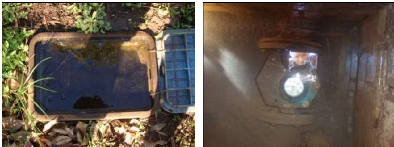
Figure 5.2: Examples of leaking domestic meters
