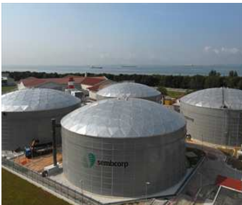
Figure 5.5 Sembcorp Changi NEWater Plant (Source: http://www.channelnewsasia.com/stories/singaporelocalnews/view/446564/1/.html )
