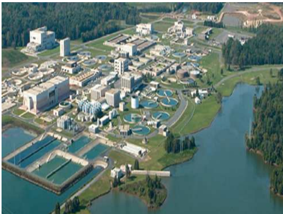
Figure 5.4 UOSA Regional Water Reclamation Plant (source: http://www.uosa-construction.org/index.asp )
