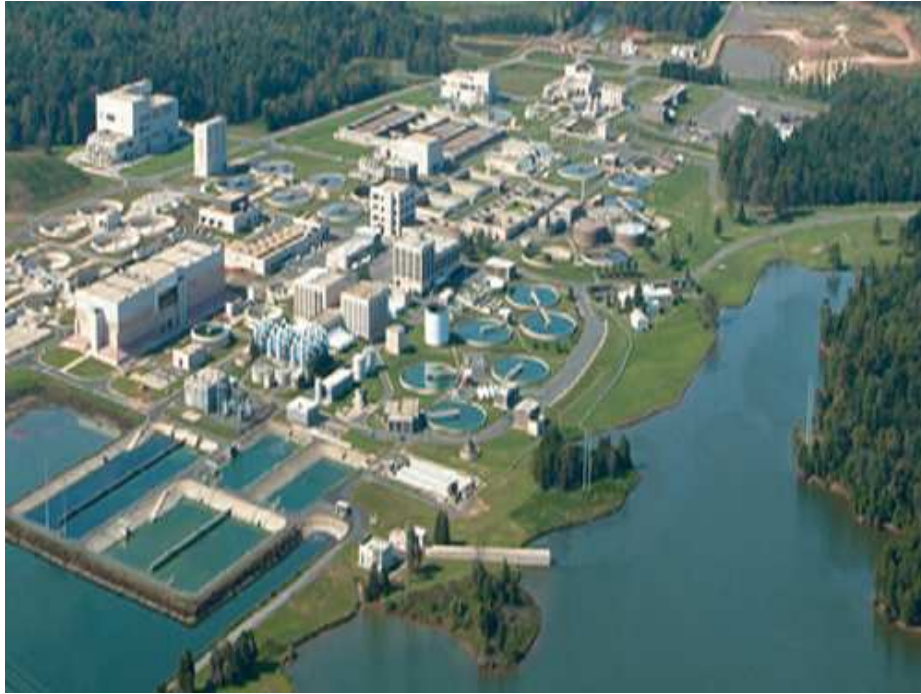
Figure 5.4 UOSA Regional Water Reclamation Plant (source: http://www.uosa-construction.org/index.asp )
