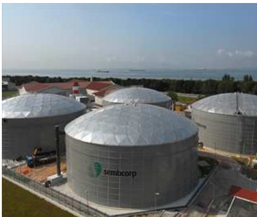
Figure 5.5 Sembcorp Changi NEWater Plant (Source: http://www.channelnewsasia.com/stories/singaporelocalnews/view/446564/1/.html )
