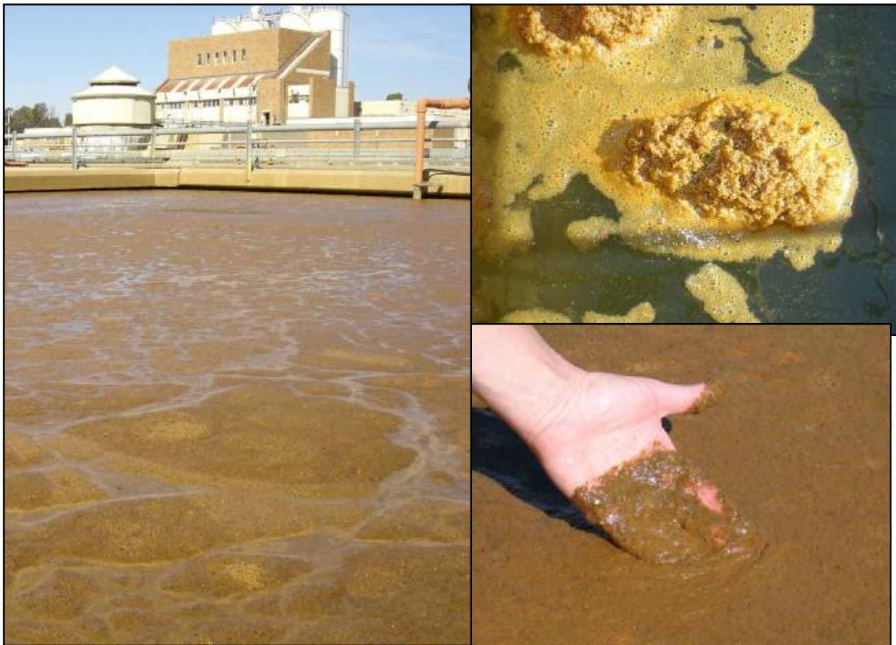
Figure 100: Thick foam scum in settling tanks of Sedibeng Water purification plant associated with a diatom ( Stephanodiscus sp.) bloom in the Vaal River at Balkfontein (3/6/2006). The dark red-brown colour is partially attributed to the diatoms and the chemicals (ferrichloride) added to the water
