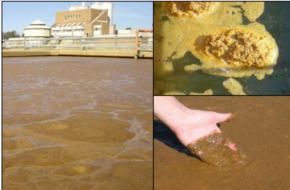
Figure 11: Thick foam scum in settling tanks of Sedibeng Water purification plant associated with a diatom ( Stephanodiscus sp.) bloom in the Vaal River at Balkfontein (3/6/2006). The dark red-brown colour is partially attributed to the diatoms and the chemicals (ferrichloride) added to the water
