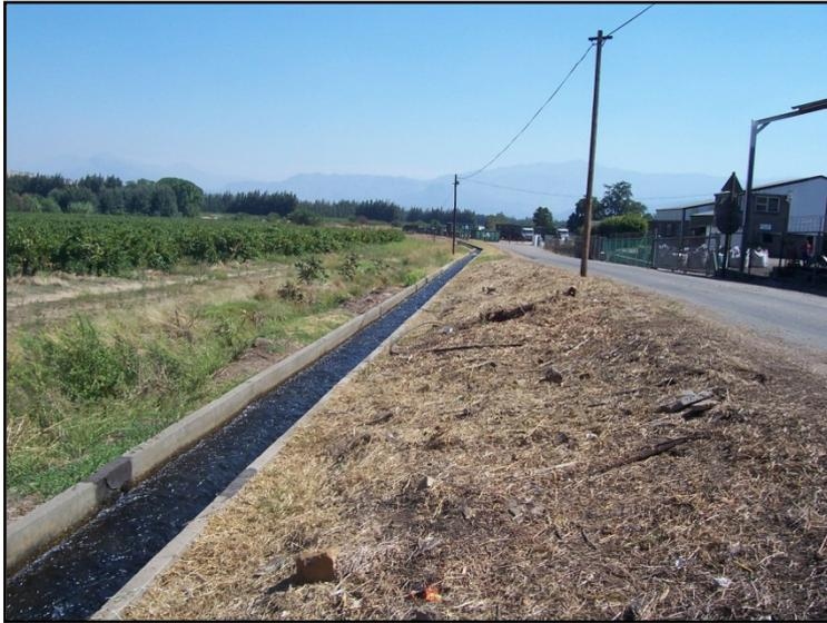
irrigation developments in the Breede River Valley, despite additional pumping to the Brandvlei Dam. Immediately downstream of the proposed scheme is the existing **Artois Irrigation Scheme**, currently reliant on diversions from the Dwars River into the Artois canal (see adjacent photograph). Ensuring ongoing supply to these irrigators (in accordance with their lawful use) will be a pre-requisite.
