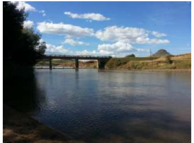
Figure 40: Downstream view of the TS6 site on the Inxu River showing the slow laminar flow at the point.
