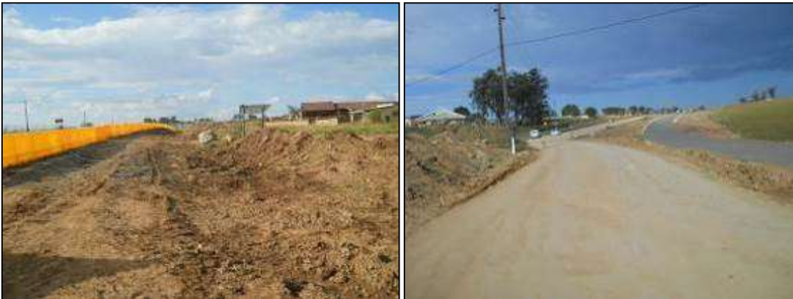
Figure 30: Current construction activities to upgrade roads outside the Qumbu area.
