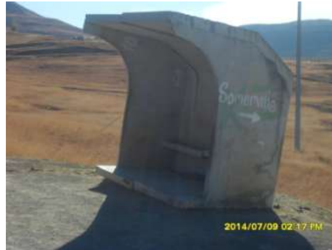
Bus stop at coordinates 31 21.7441S 28 62.4328E
