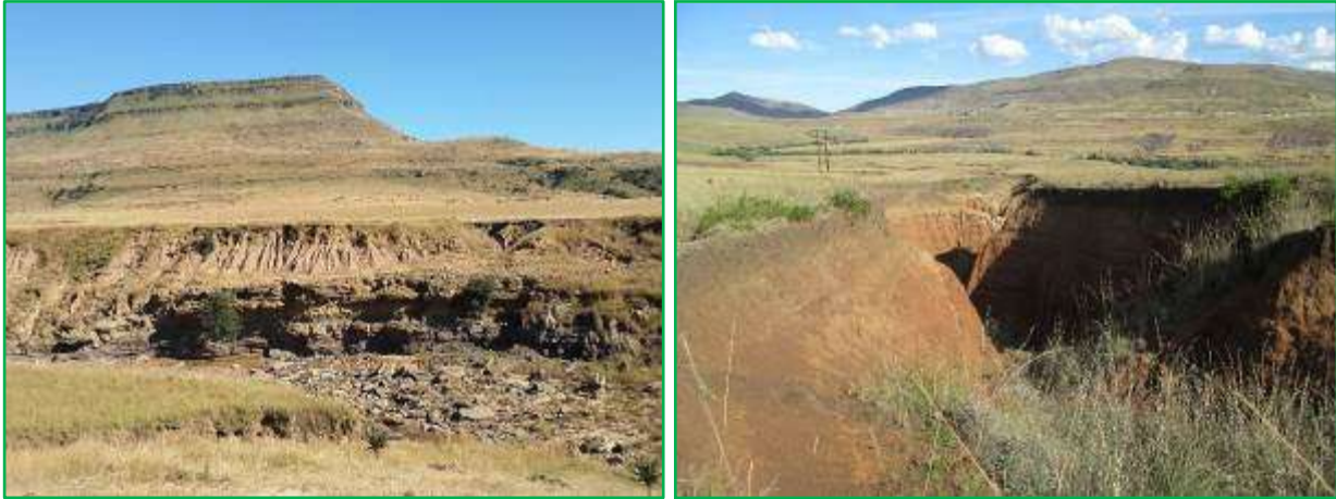
Figure 12: Representative photographs showing examples of the typical erosion patterns within the catchment.
