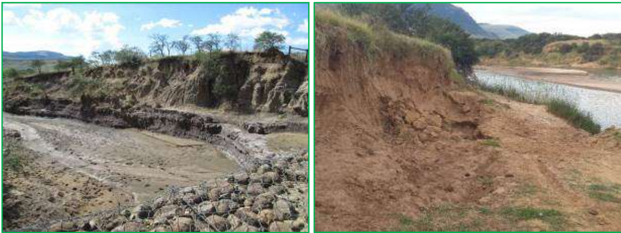
Figure 11: Representative photographs showing severe incision and erosion of river banks (left) and sediment winning (right).
