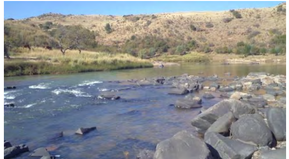
Figure 20: A downstream view of the TS4 site in the vicinity of the proposed Ntabelanga dam wall, as assessed in June 2014.
