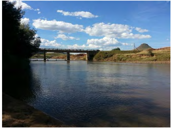
Figure 40: Downstream view of the TS6 site on the Inxu River showing the slow laminar flow at the point.
