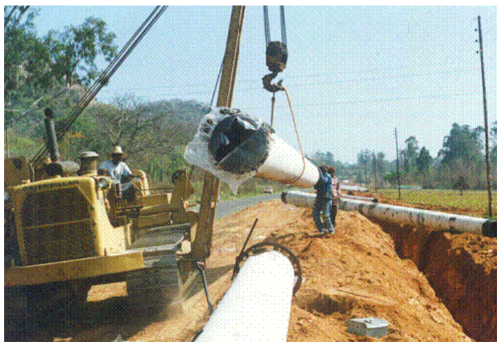
Figure 16: Trench and working area for pipe lying
