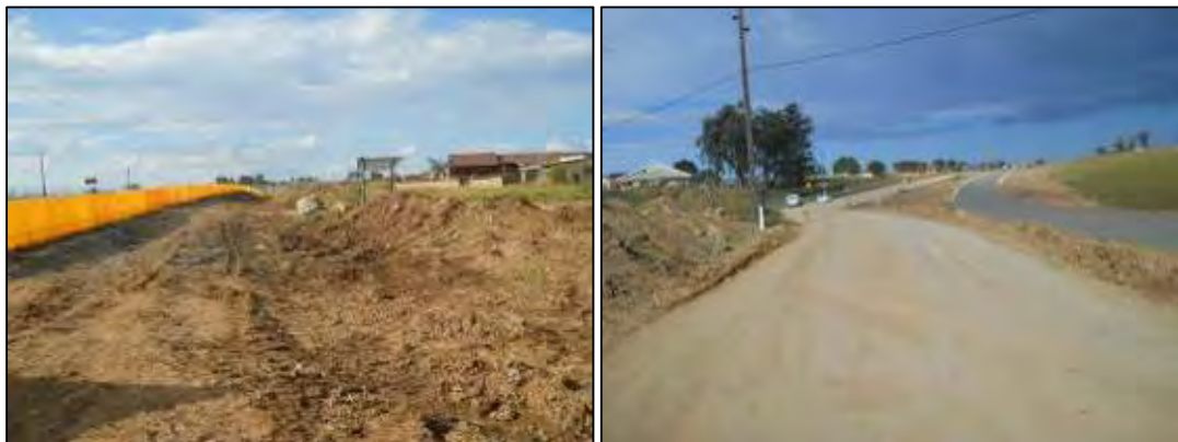
Figure 30: Current construction activities to upgrade roads outside the Qumbu area.
