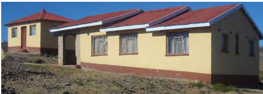
Figure 36: Indirectly affected dwelling at coordinates 31 27.6635S 28 95.2361E
