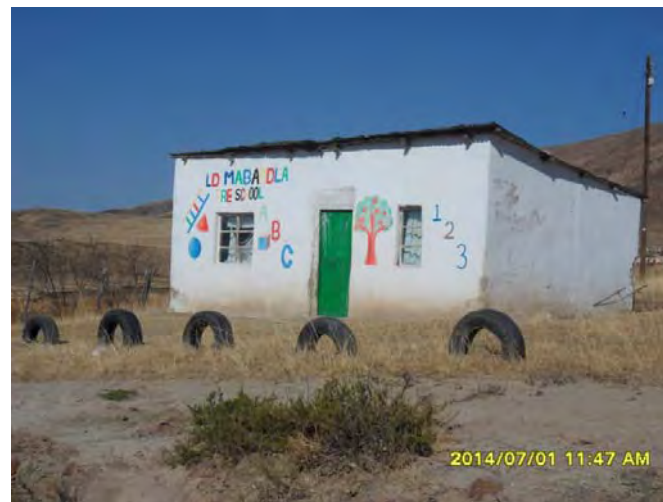
Pre-school at coordinates 31 12.5844 S 28 65.7729E
