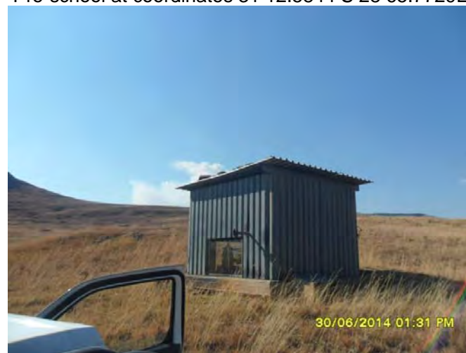
Water pump at coordinates 31 08.8654S 28 66.0927E
