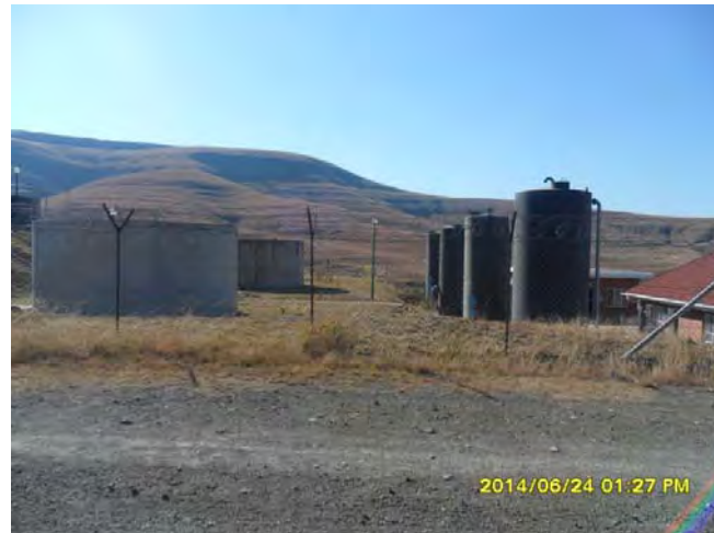
Water purification plant at coordinates 31 08.5436S 28 61.9594E
