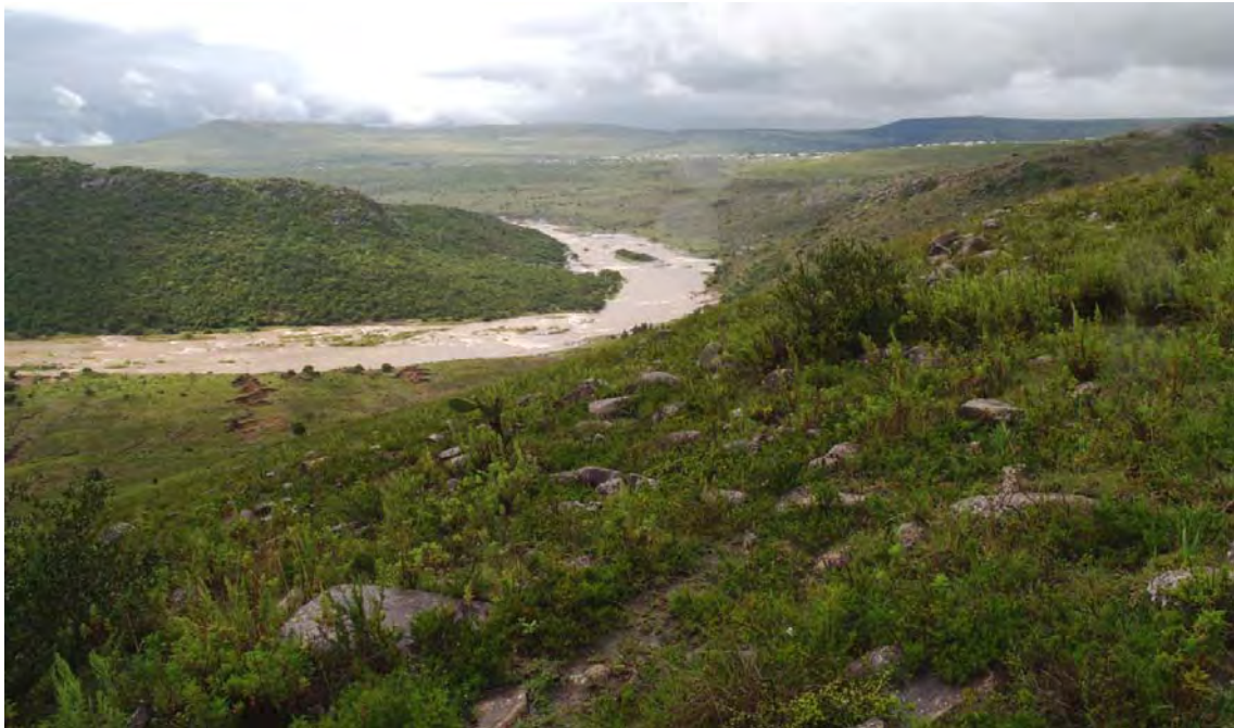
Photo 2: Dam wall site for the Lalini Dam
