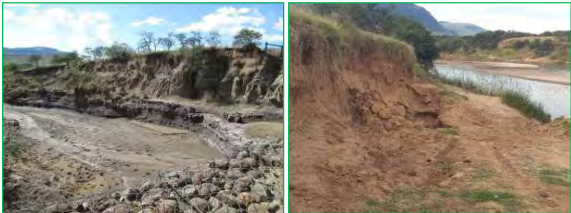
Figure 11: Representative photographs showing severe incision and erosion of river banks (left) and sediment winning (right).
