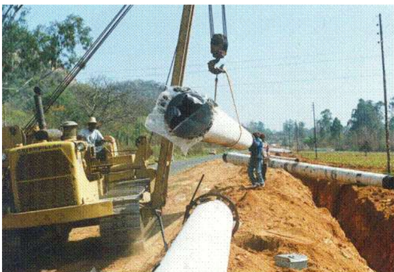
Figure 16: Trench and working area for pipe laying
