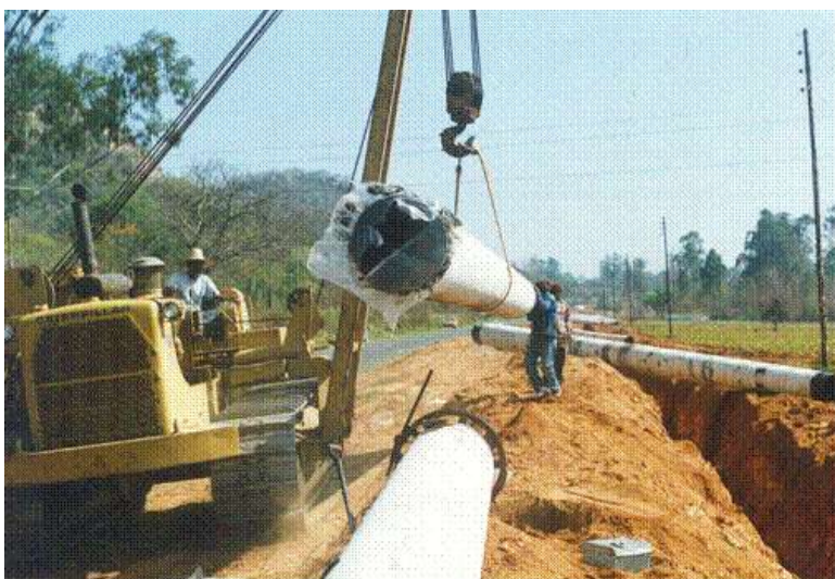
Figure 16: Trench and working area for pipe laying
