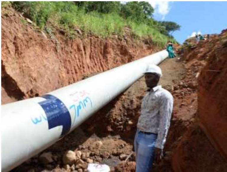
Figure 15: Pipe laying
