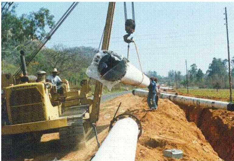
Figure 16: Trench and working area for pipe lying
