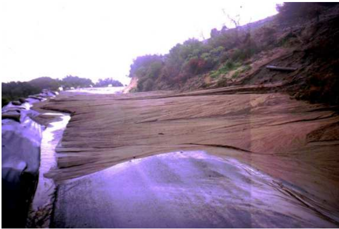
Massive sediment deposition on Chapmans Peak drive above Noordhoek, 31 May 2000, four months after the fire. Alien and cleared vegetation occurred above this site.
